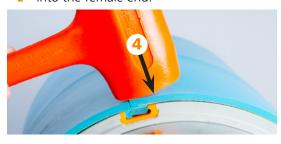
When properly installed, the lockup area should be smooth and even with no steps.
